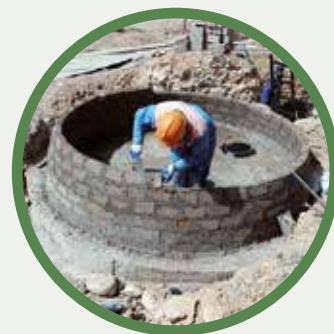
Construction of the fixed-dome type agricultural digester in the village Ait Idir.
