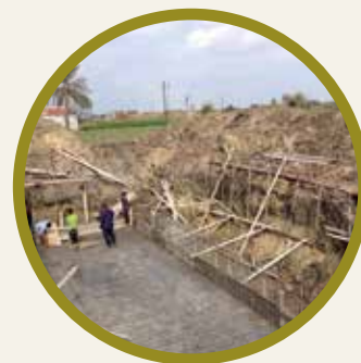
Construction of the compact treatment plant.
