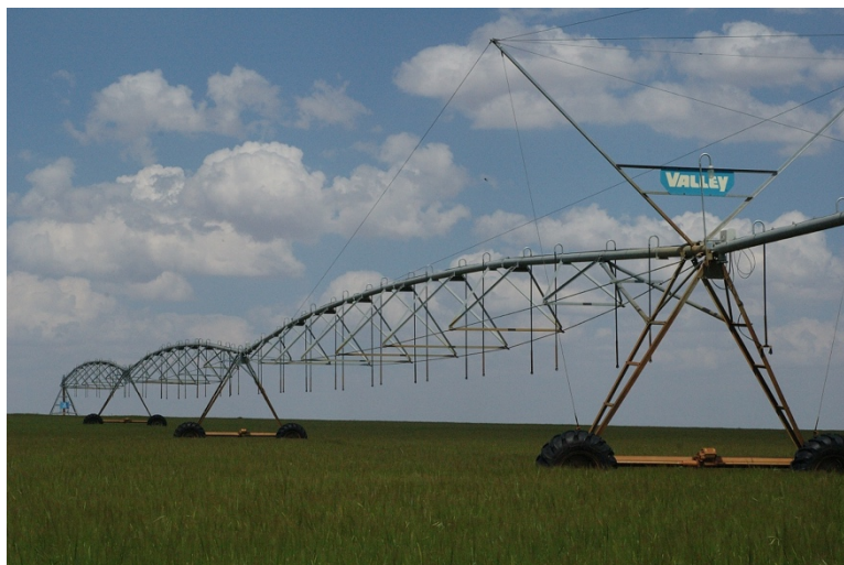
Figure 10 - Irrigation system in Daimel, Spain Photo Credit: Jan van der Straaten
